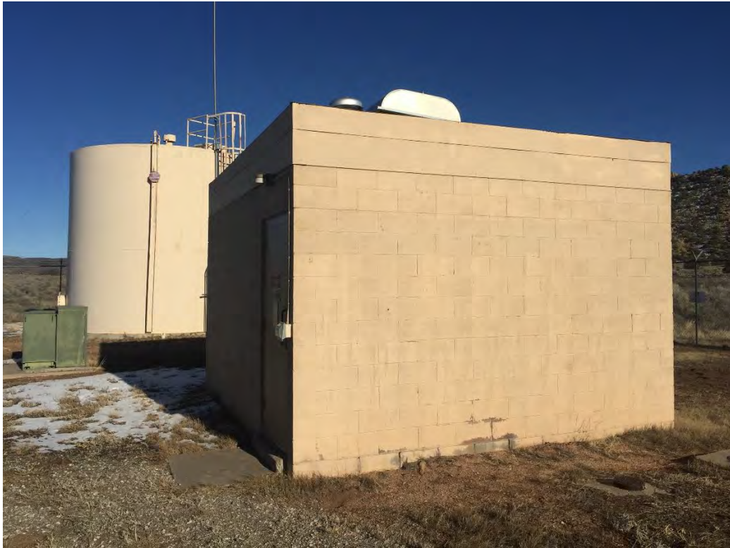
Figure D10. Well 9 BPS and Tank
