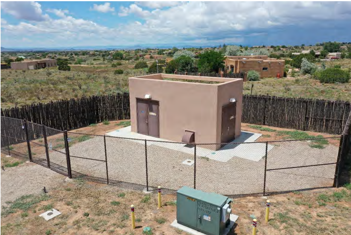
Figure D2. Torreon Booster Pump Station
