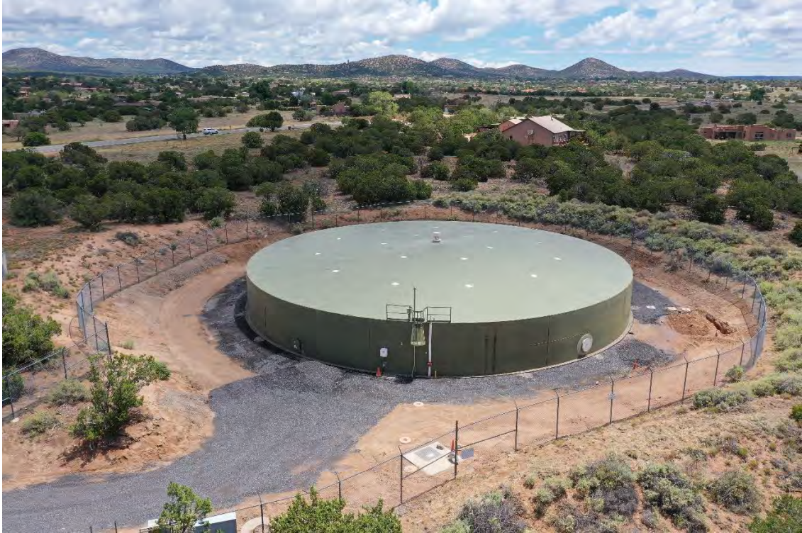
Figure D7. Tank 4
