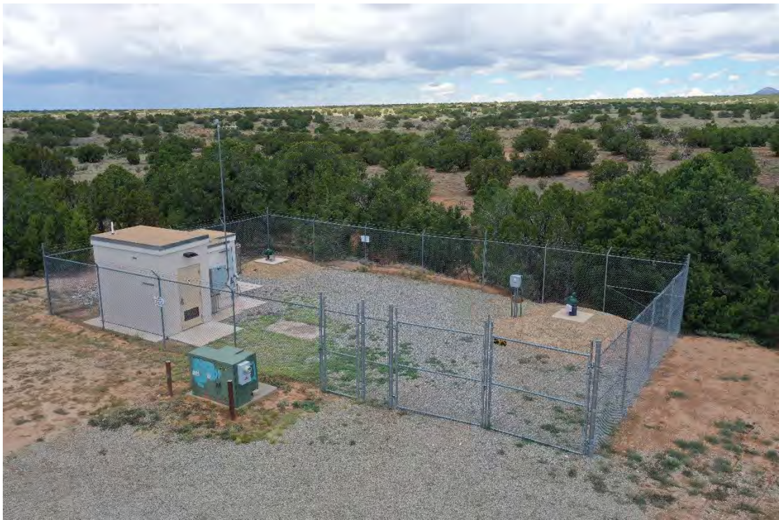
Figure D8. Well 2A-2B
